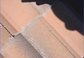
3.2 Although there are no apparent deficiencies with the roofing material, there are moisture stains within the residence that we will identify. However, active leakage can be difficult to trace and confirm when it is not raining, a roofing specialist should further evaluate and repair as needed..
